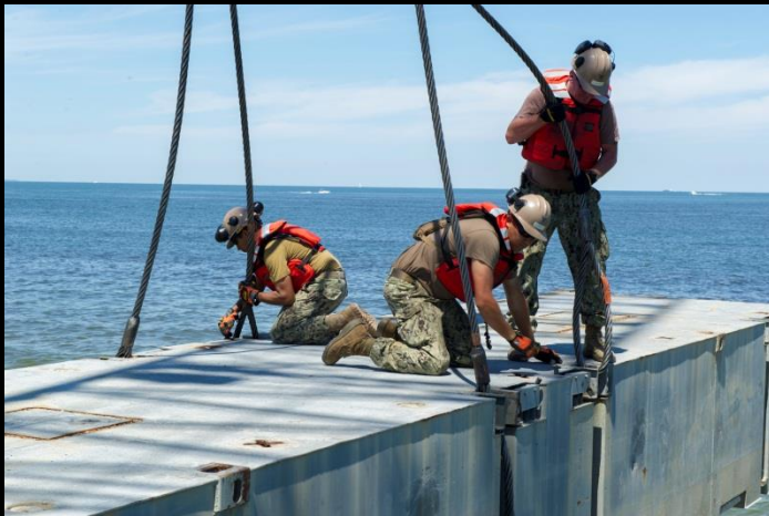
Active and Reserve Seabees assigned to PHBCB TWO and PHBCB ONE construct the Elevated Causeway System (ELCAS) onboard Joint Expeditionary Base Little Creek. (U.S. Navy photos by Engineering Aide 2nd Class Larry Winer)
