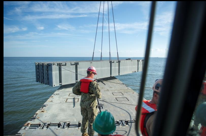
Active and Reserve Seabees assigned to PHBCB TWO and PHBCB ONE construct the Elevated Causeway System (ELCAS) onboard Joint Expeditionary Base Little Creek. (U.S. Navy photos by Engineering Aide 2nd Class Larry Winer)
